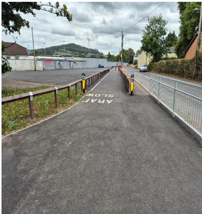
Widening of the footpath near the school on Pen-y-Pound
