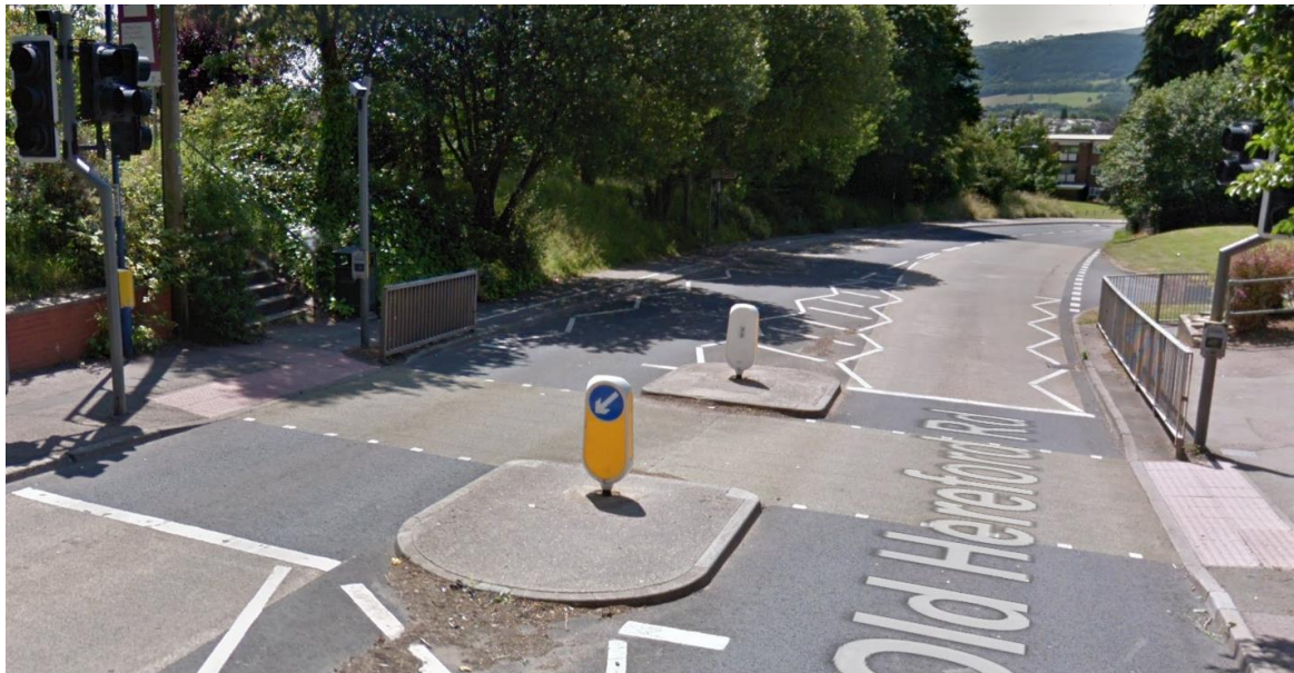
Footpaths on both sides of the road and dropped kerbs and tactile paving at the crossing point
